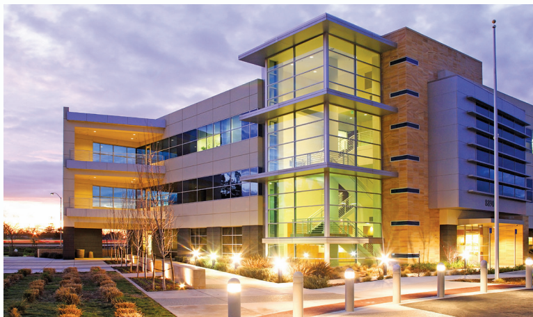
LARGE HVAC APPLICATIONS
