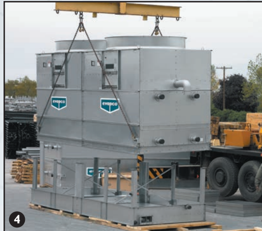
4 Mount Fill or Coil/Fan to Basin Section
