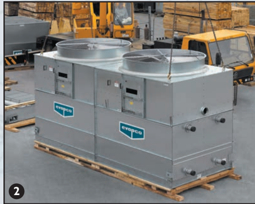
2 Mount Fan Section to Fill/Coil Section
