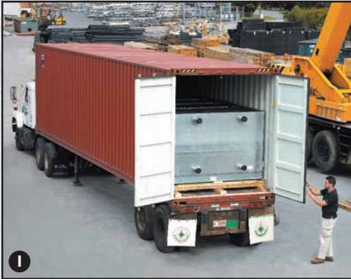
1 Unload Unit from Container
